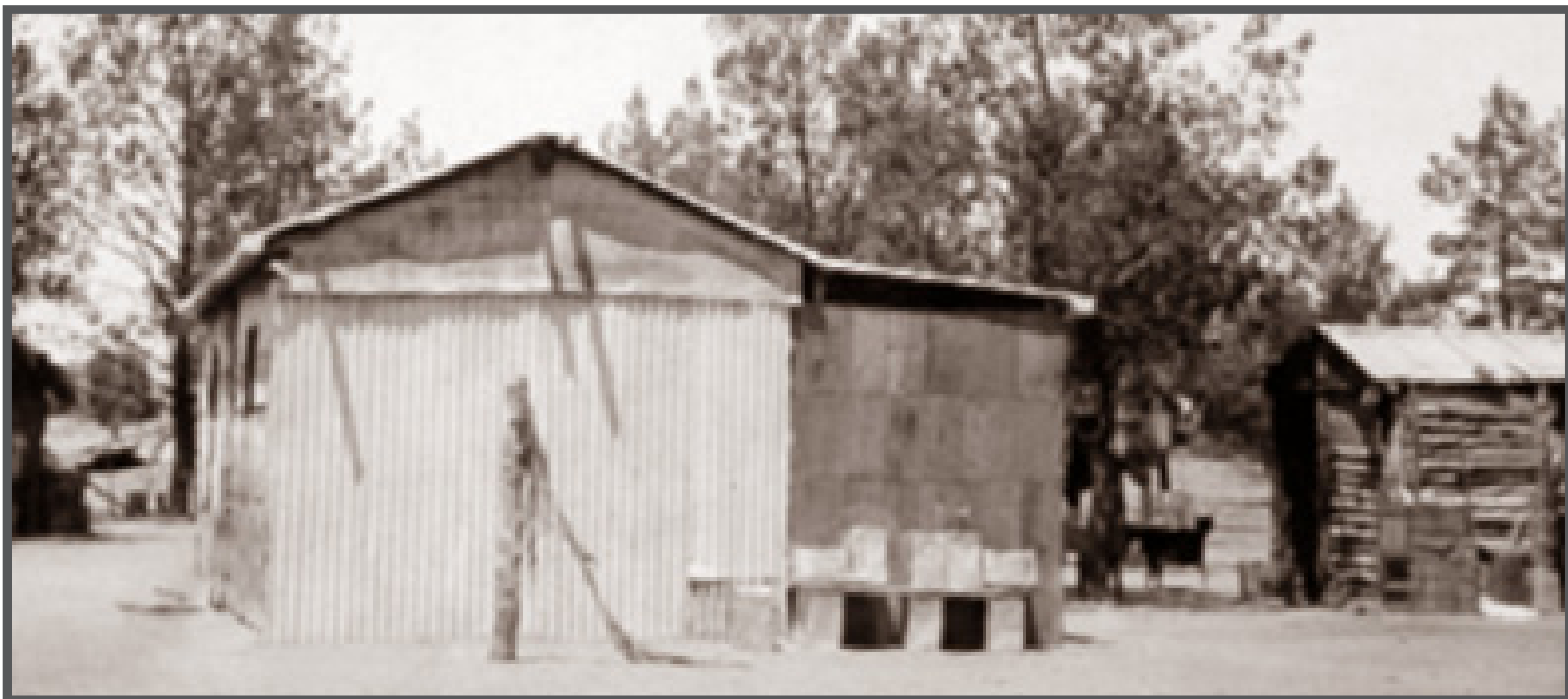
The original "Zanci" homestead circa. 1925 was built from iron and flattened kerosene tins. It had 2 rooms, and a small drop log kitchen (in right of photograph).
