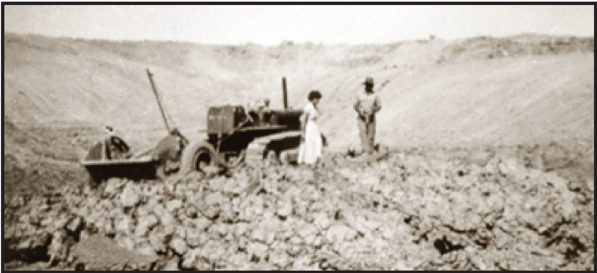
Below: Albert and Venda Barnes in the process of enlarging the Scour Tank to serve as the main house tank with TD9 tractor.
